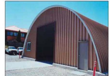
After all panels are welded or fastened to the foundation steel, the end cap is set, and concrete is poured.
